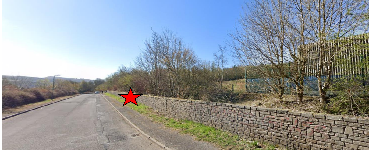
Red Star indicates approximate position of access to be created off Gwent Way
