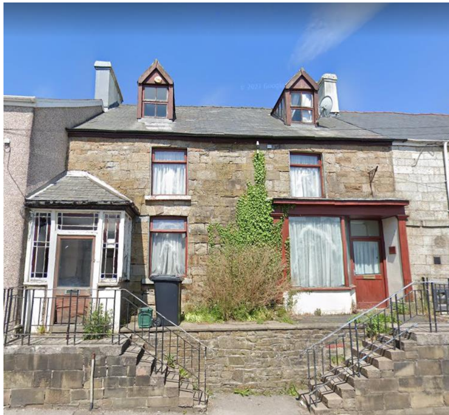
Fig. 1.1 Existing Property at 74 A King Street
