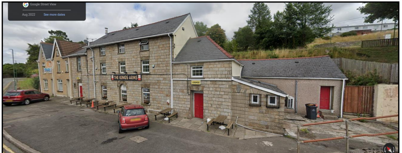
Image 1- Street view image of application site from Newchurch Road with adjoining dwellings finished with buff coloured render.
